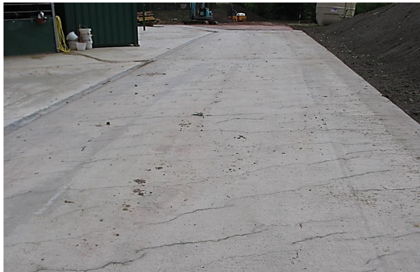
Figure 2: Shrinkage cracking in rigid pavement
