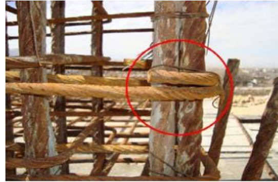
Figure 2: Bent Reinforcement and Non-Seismic Hooks
