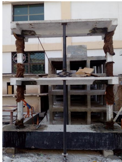
Figure 2: Removal damaged concrete. Figure 3:
