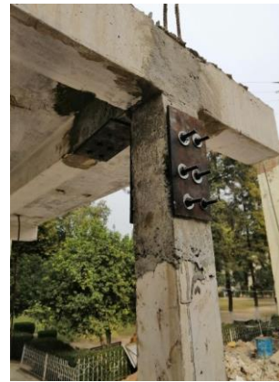
Figure 6: Through Anchorage in beam and columns
