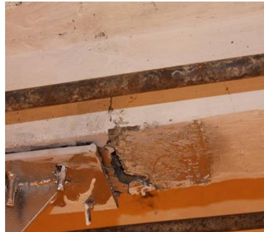
Figure 7: Flexure cracking in beam of retrofitted frame.
