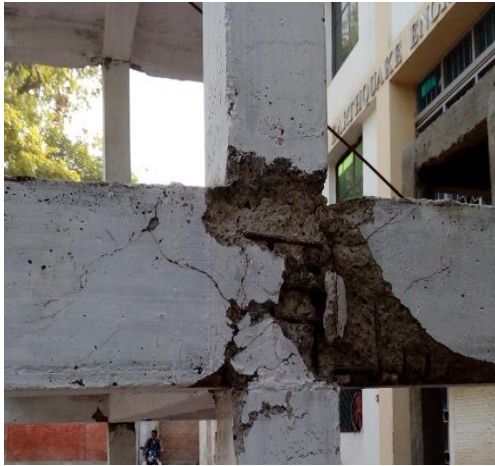
Figure 6: Damage in joint of as-built frame
