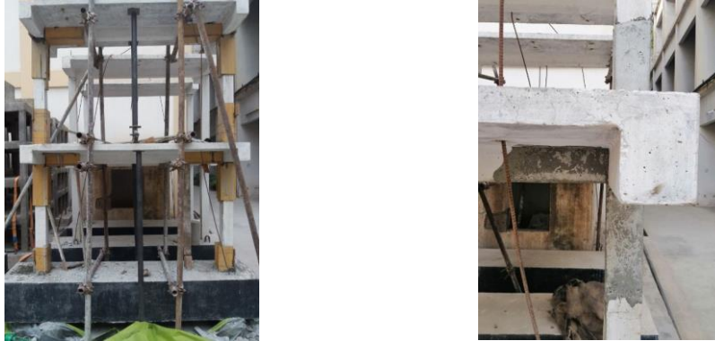
(d) Formwork for concreting, (e) Joint after replacing damaged concrete
