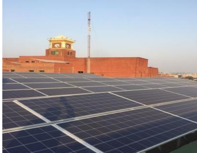
Figure 5: Solar panels installed on roof.
