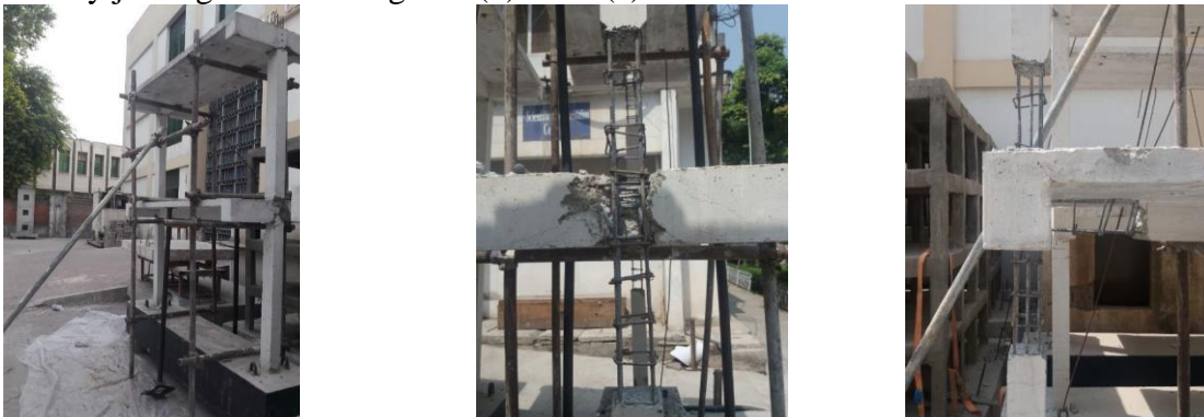
Figure 3: (a) Damaged Frame, (b) Damaged concrete removed from joints, (c) Joint after concrete removal
